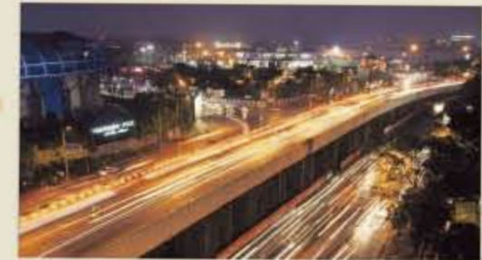
Eastern & Western Express Highways (Upcoming Eastern Freeway)
